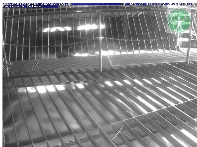
Tunnel inlet at capacity during high flows
