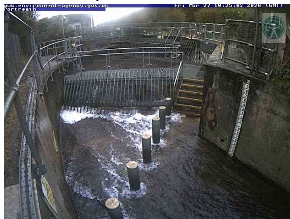
Tunnel entrance during normal flows
