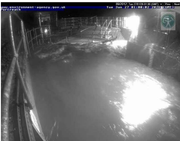
Tunnel entrance during high flows
